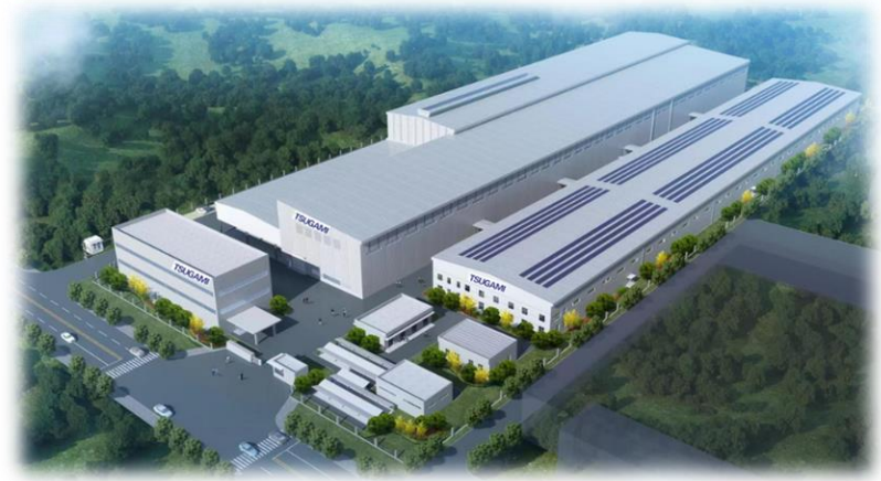
Rendering of the plant after renovation
